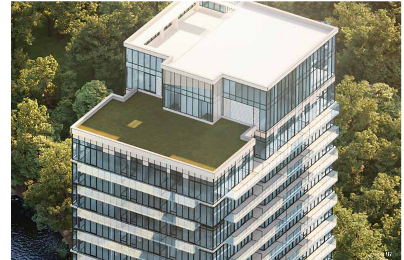
Green roofs absorb rainwater and reduce energy consumption
